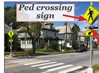
Pedestrian crossing sign & flashing lights (RRFB)
